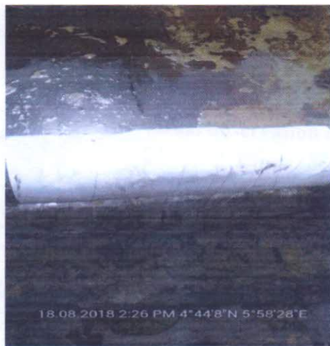
Fig C: picture taken after wrapped.
