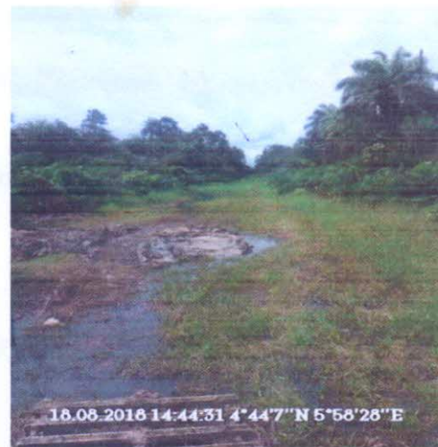
Fig D: picture taken after backfilled.
